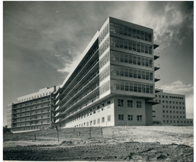
Finishing up construction of Van Etten Hospital
